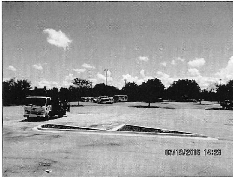
Parking lot area in front of the building.
